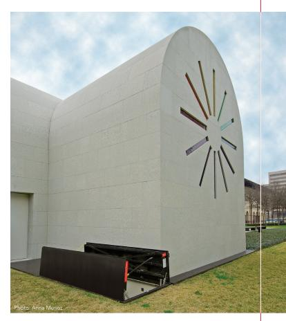
less noticeable from the exterior and a keyed cylinder lock for added building security. The large custom door sits on the outside of the structure, next to one of only two emergency exits in the building and features BILCO's engineered lift assistance for one-hand operation. "Many people don't even know where there is access to the basement," Lancaster said. "We had to have access to the basement, but we also had to make the door, as much as we could, invisible."
